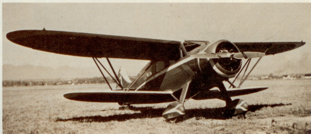
A UKC seaplane of the 1934-1936 era. Note additional fin area added under the fuselage for seaplane operation. On some Wacos, pronounced WAH-cos, a wide fairing on the diagonal of the N-strut could be turned 90 degrees to the airstream to act as a small air brake. Photo by Robert Esposito
